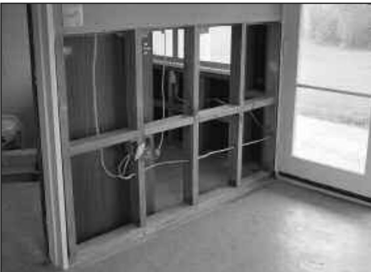
Figure 3. Floor coverings and wall linings have been removed to allow the framing to dry.
