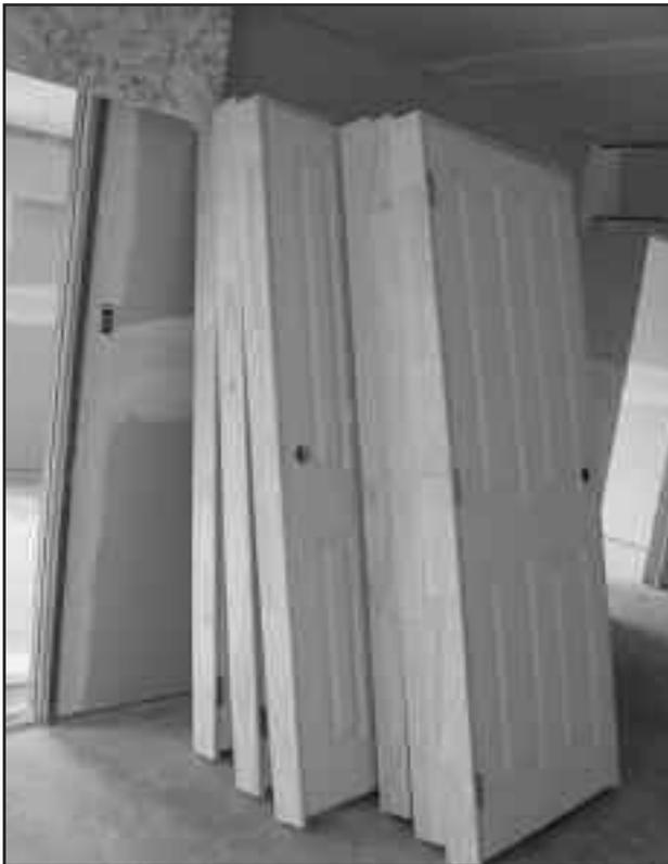
*Figure 5. It is probable that new doors and frames will be needed if the water immersion has been anything other than brief.*
