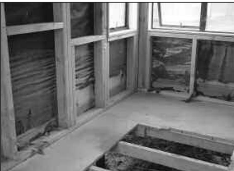
Figure 2. This building paper will need replacing necessitating the removal of the exterior cladding.
