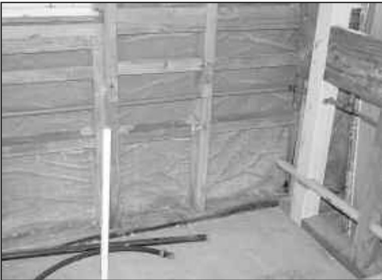
Figure 1. The building paper should be inspected closely for damage and the framing condition and treatment determined.
