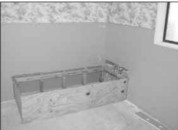
Figure 4. In this instance a full sheet width of plasterboard has been replaced and the bath framing renewed.
